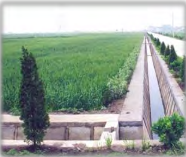
Canal lining in Shaanxi
