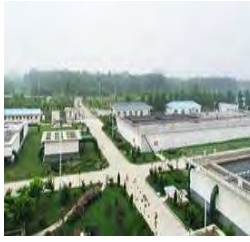
Bio-Dopp process in Chengbei WWTP
