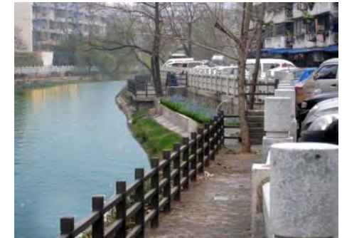
Ecological embankment for purifying runoff in Qinhuai river
